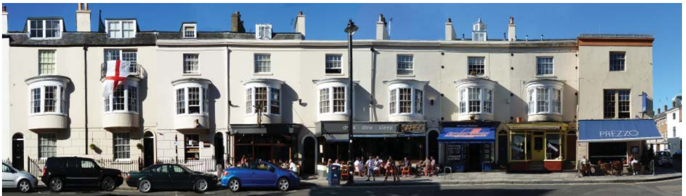
17 Oxford Street Grade II Listed
