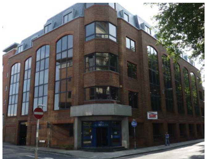
Late-twentieth century office block on a prominent corner by Queen's Park
