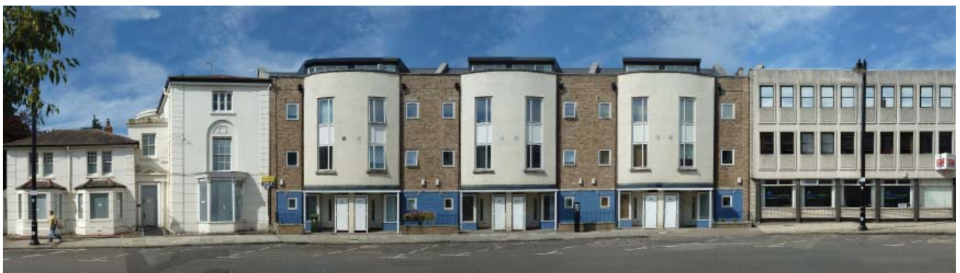
61 Oxford Street Grade II Listed
