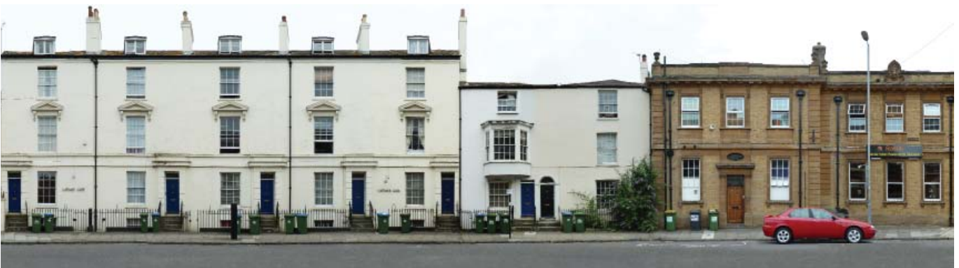
10-1 Latimer Gate, Bernard Street Grade II Listed
