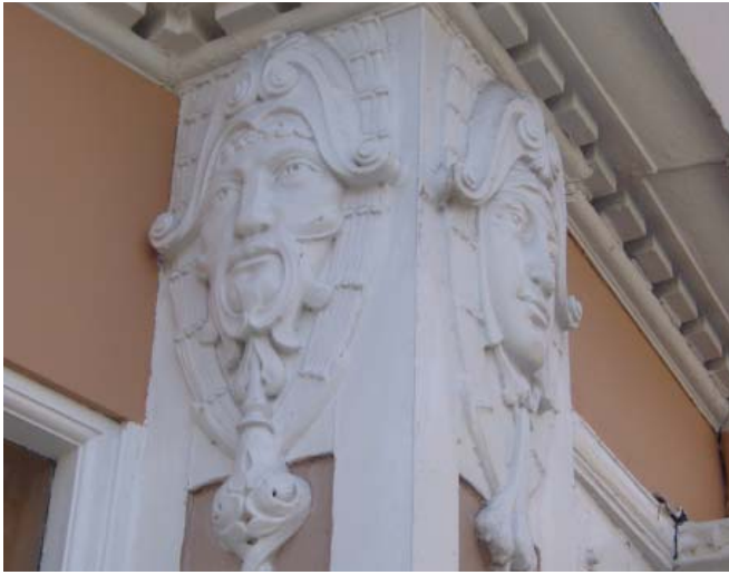
Decorative mouldings, 48-49 Oxford Street
