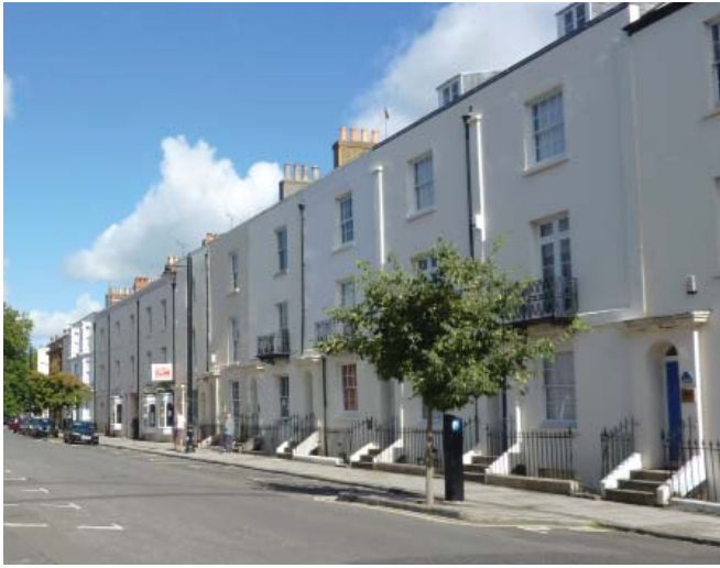
Early-to-late nineteenth century town houses, some converted to shops, Oxford Street
