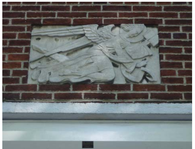
Detailing on The Southampton Seafarer's Centre, 12-14 Queen's Terrace
