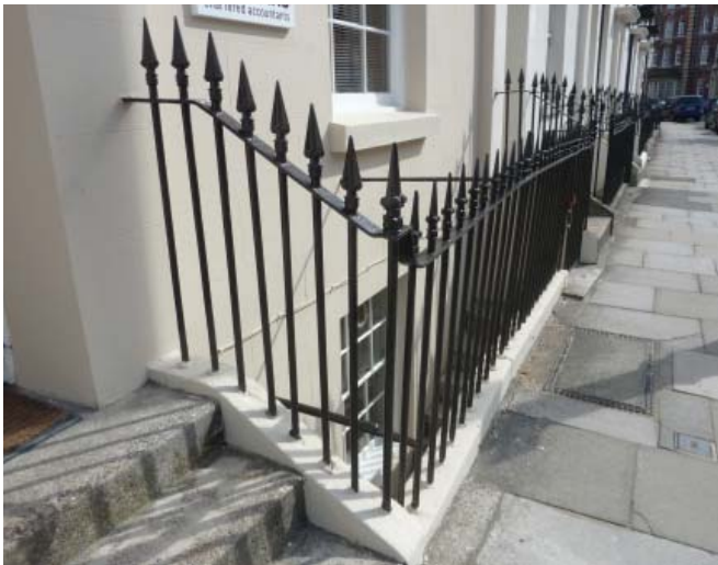
Attractive cast iron railings with spear heads defining the threshold to the property, Oxford Street
