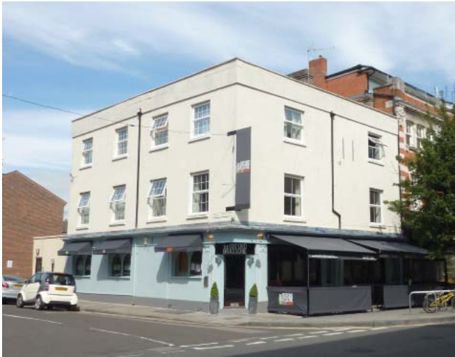
Simple stuccoed corner building, undermined by the insertion of uPVC windows, Oxford's Brasserie, Oxford Street
