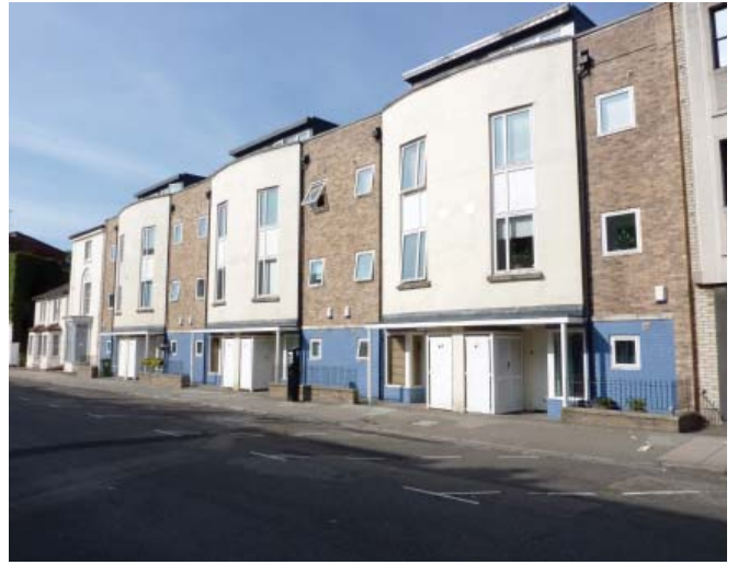
Twenty-first century infill housing, 62-65 Oxford Street
