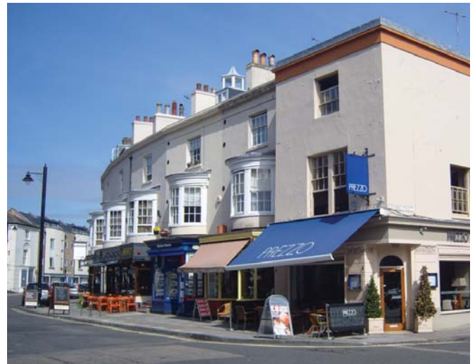
Mixed uses on Oxford Street
