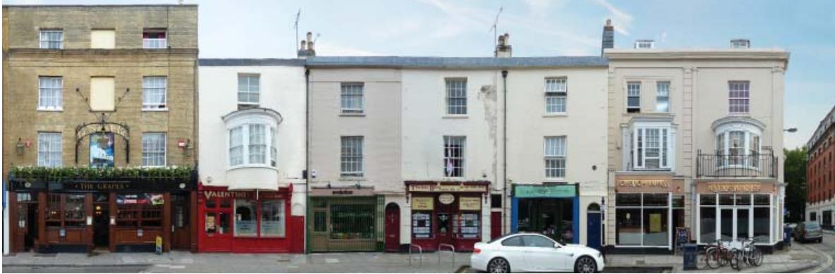
41-43 Oxford Street Grade II Listed
