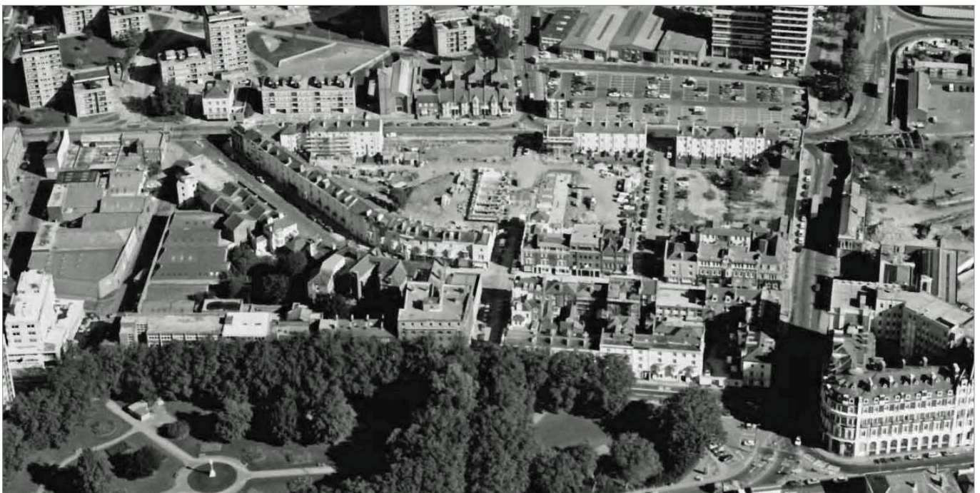
Figure 20: Extensive demolition in the Conservation Area 1970s -1980s
