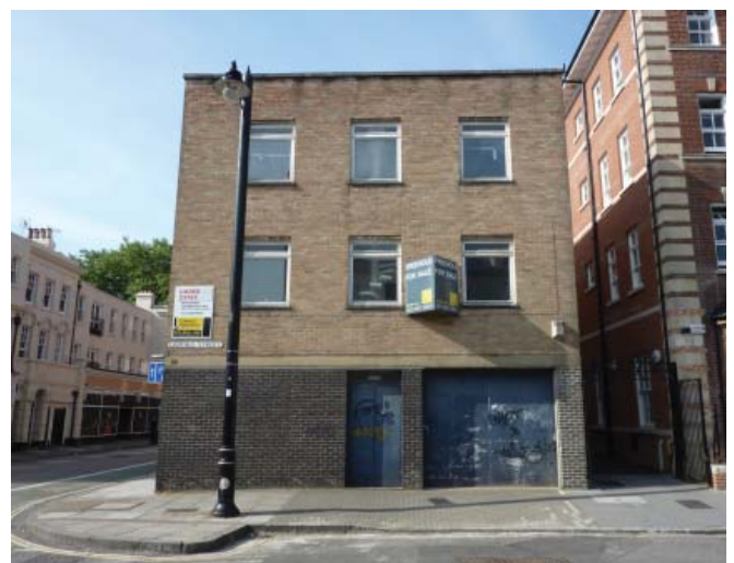
Vacant building in a prominent corner, Oxford Street
